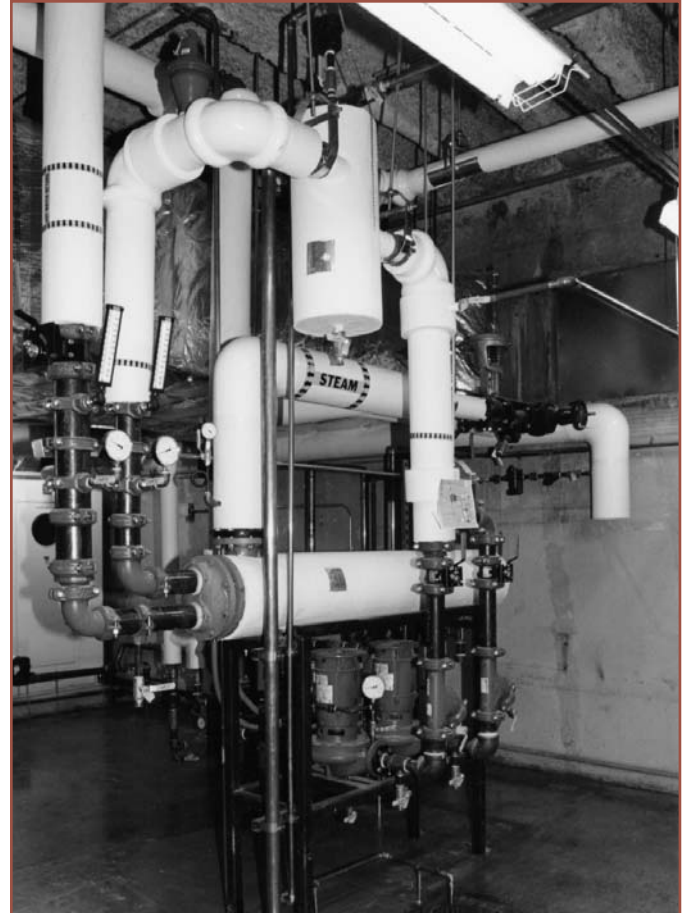
B&G inline pumps and Triple Duty® Valves
