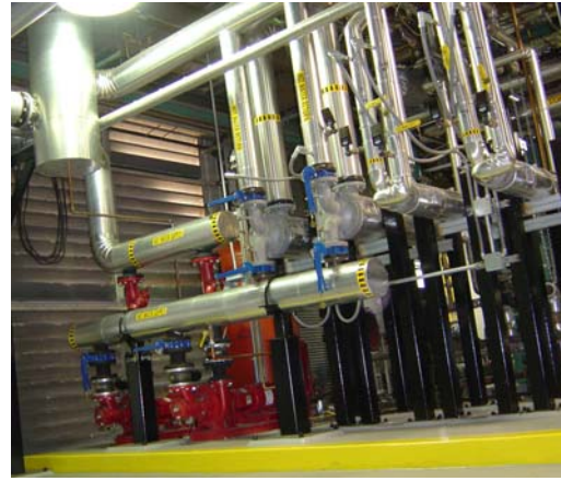
BELL & GOSSETT Hot water pumps, shell and tube heat exchangers, air separator
